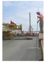
Trapped water/air and elongation of air voids typically occur when finishers apply a finish to the slab before all the bleed water can reach the surface. It can also occur when the ambient conditions of temperature, wind, and humidity result in a high evaporation rate for the bleed water, which causes premature drying and stiffening of the near-surface layer and traps bleed water and air below the surface.
